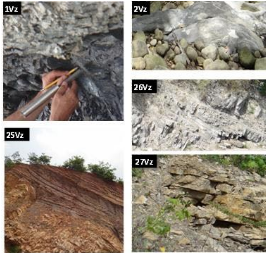
Figure 5.37. Sampled sites in the East of the Urica Fault (Bergatín Block in the Serranía Del Interior)
